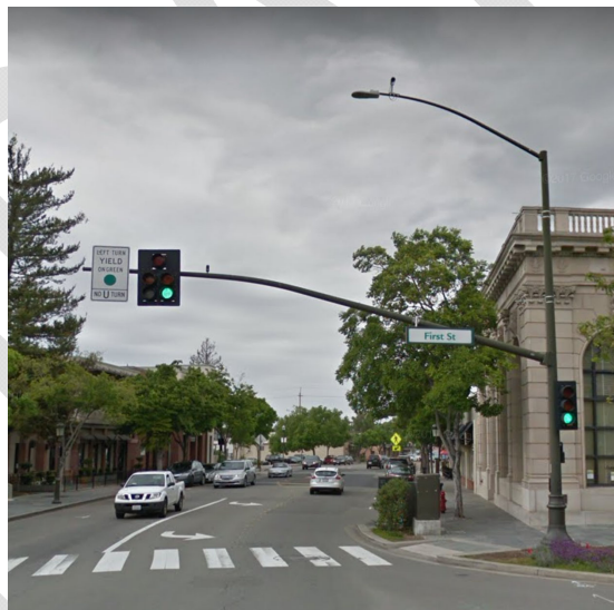
Figure 1-2 Traffic Signal Pole/Street Light Example
